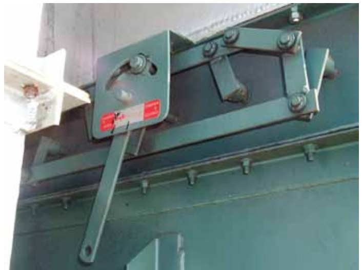
FIGURE 2. FAN DAMPER WITH POSITION MARKS INDICATING CALIBRATED AIRFLOW
